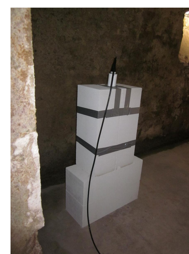
Fig. 4: A Caesium-magnetometer in Graz. The locations for each of the stations were suggested and evaluated by students. This station is in a private cellar. The station in Tamsweg was set up in the school, while the station in Innsbruck was formerly in a tunnel on the city outskirts.
